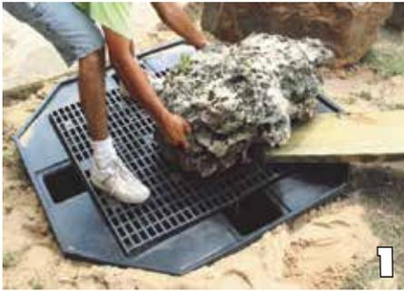
1. Carefully set feature in center of grating\*. Align hole in feature with hole in grate. It may be necessary to cut a larger hole in the grating to accommodate bigger tubing.
