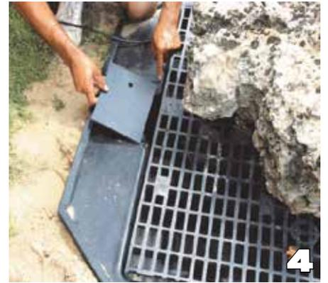
4. Place lid over pump compartment. Spread decorative gravel or river rock on grating, just enough to cover grating is all that is required. You can easily remove the pump anytime by clearing the gravel or river rock off lid. Fill basin with water and plug pump into a GFI protected outlet with weather cover.
