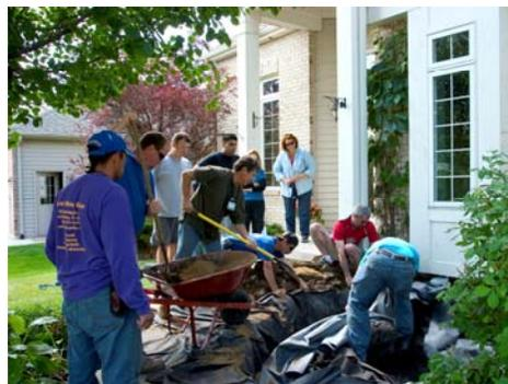
Liner is spread before the AquaBlox® D-Raintanks® are placed.
